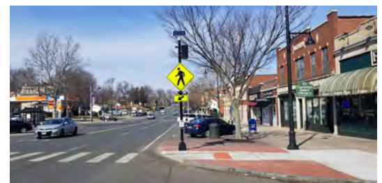
Rectangular Rapid Flashing Beacon (Main Street)
