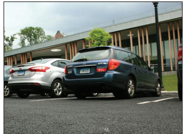
Figure 4. Pervious asphalt on the UConn campus in Storrs, CT.
