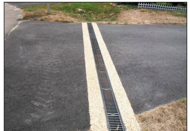
Figure 1. Trench drain in residential driveway.
