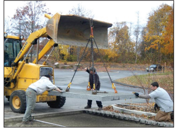
Figure 6. Precast pervious concrete panels being installed in East Lyme, CT.
