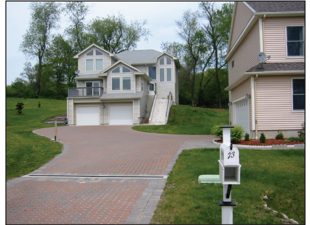
Figure 3. PICPs on a residential driveway in Waterford, CT.
