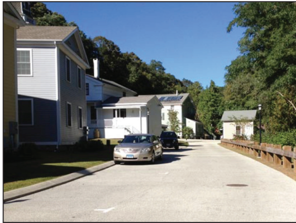
Figure 5. Pervious concrete installation in East Haddam, CT.
